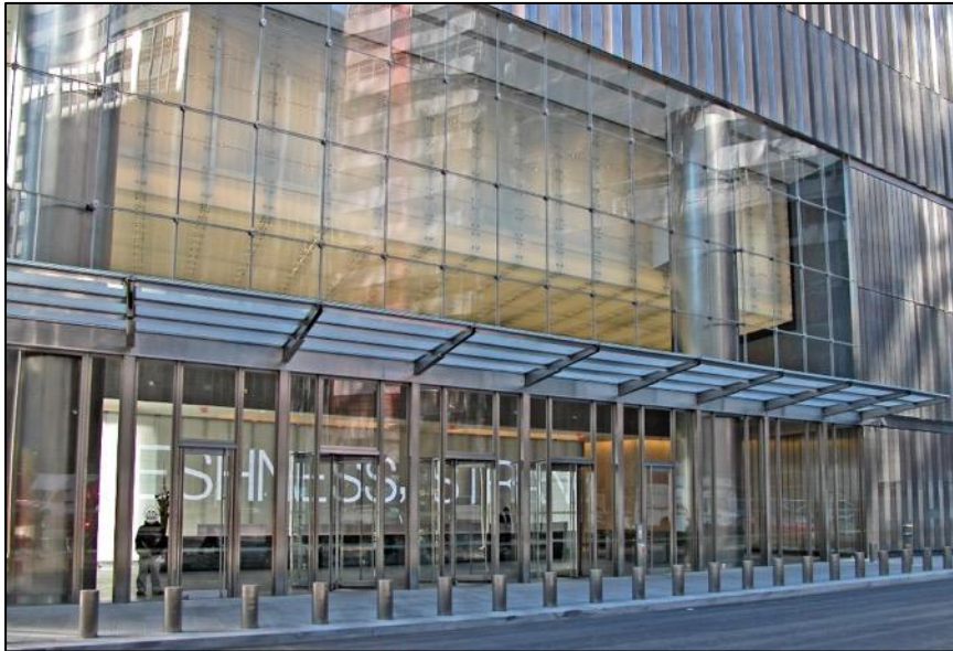
Stainless steel columns, entrance canopy at Seven World Trade Center, New York
